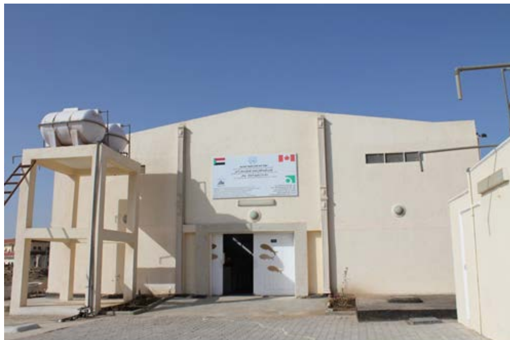
The Landing site constructed at Suakin
